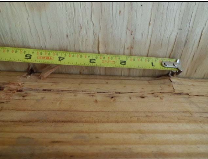
Roof deck attachment
