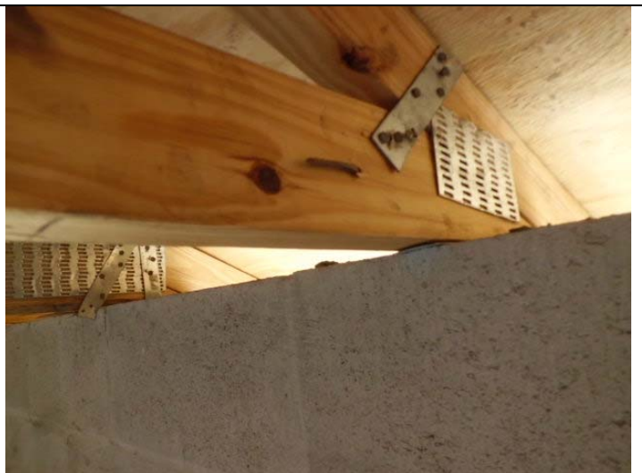
Roof to wall attachment
