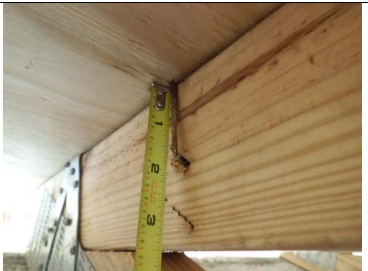
Roof deck attachment
