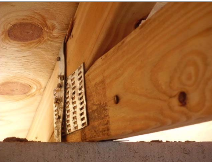
Roof to wall attachment
